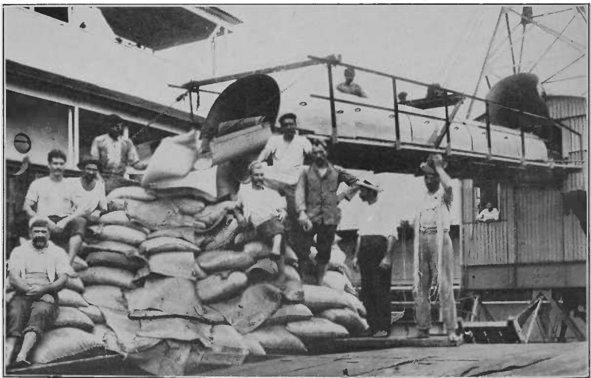
DELIVERY OUTLET OF THE ENDLESS RUBBER CONVEYOR OVER THE SHIP'S HOLD
