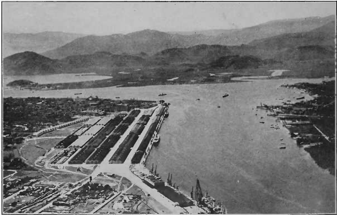
BIRD'S-EYE VIEW OF THE NEW COFFEE WAREHOUSES
