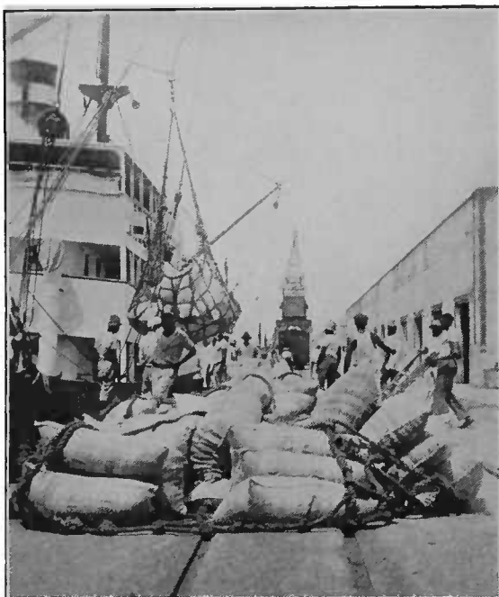
NETS CARRYING TWENTY-FIVE BAGS ARE USED FOR LOADING COFFEE AT BUENAVENTURA
