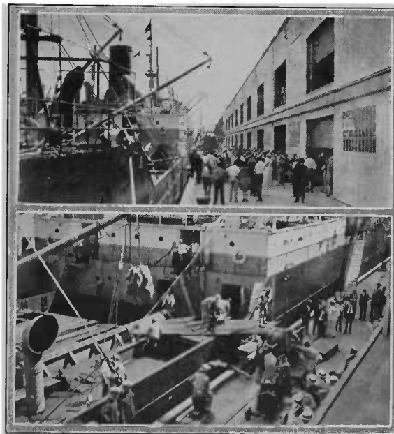
COFFEE UNLOADING SCENES AT NEW ORLEANS Upper —Showing the relative positions of dock and storage sheds. — Lower —Unloading coffee into trailers for transportation to shed.
