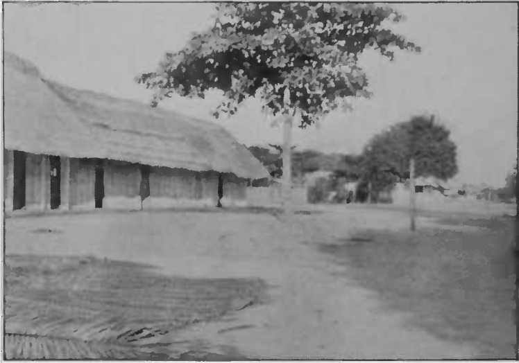
THE FRONT STREET OF CONTAMANA. NEW THATCH DRYING IN THE SUN
