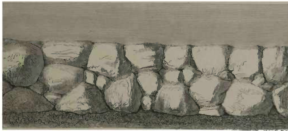
CYCLOPEAN CONSTRUCTION IN THE LATER PERIOD OF THE INCAS.
