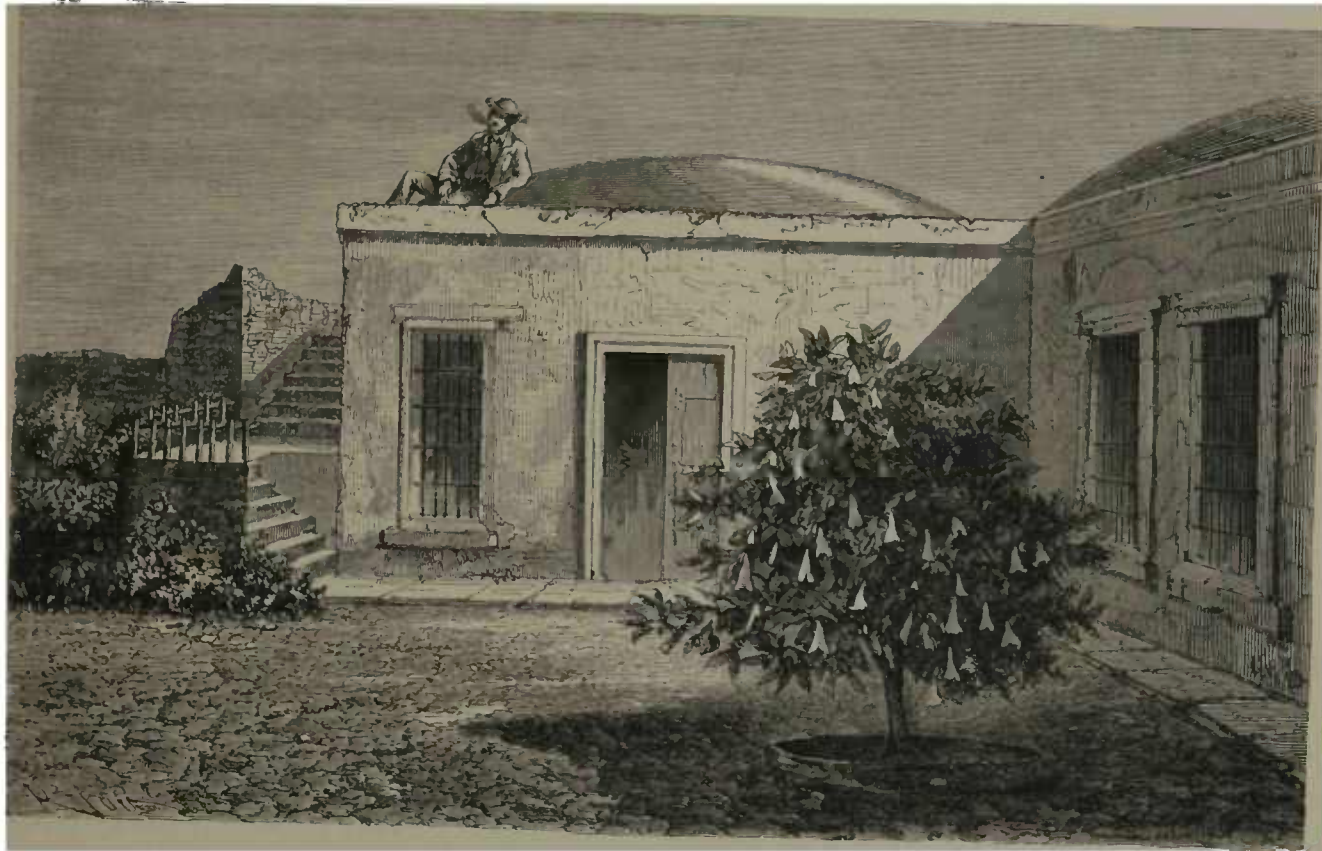
THE AUTHOR'S HOUSE AT AREQUIPA.
