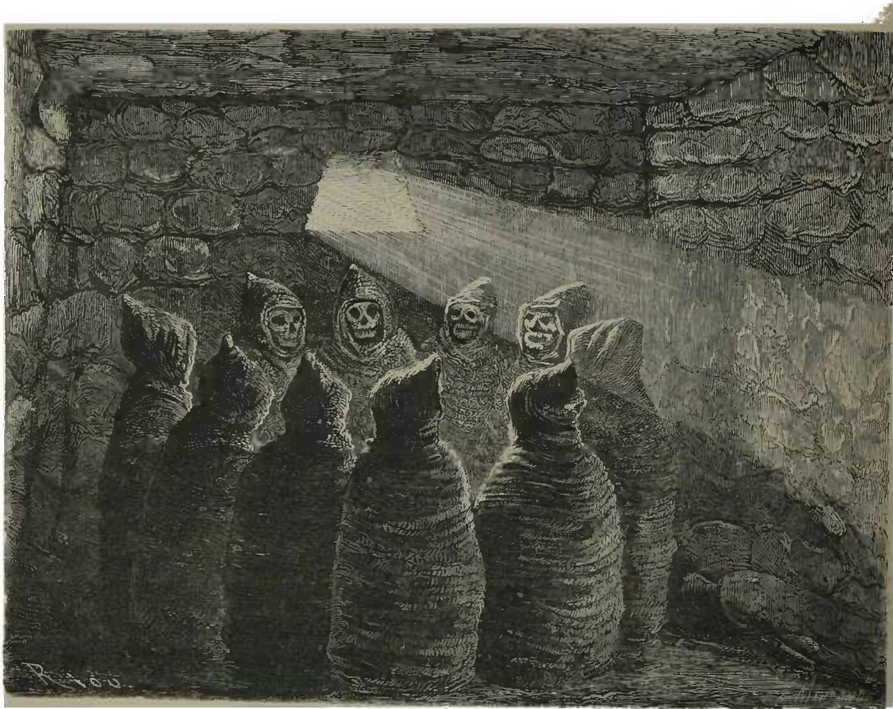
INTERIOR OF AN AYMARA CHULPA.
