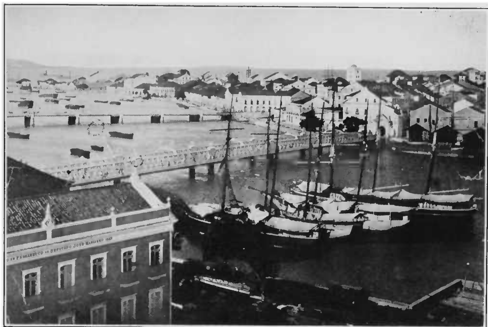
A Partial View of the Business District of Pernambuco.
